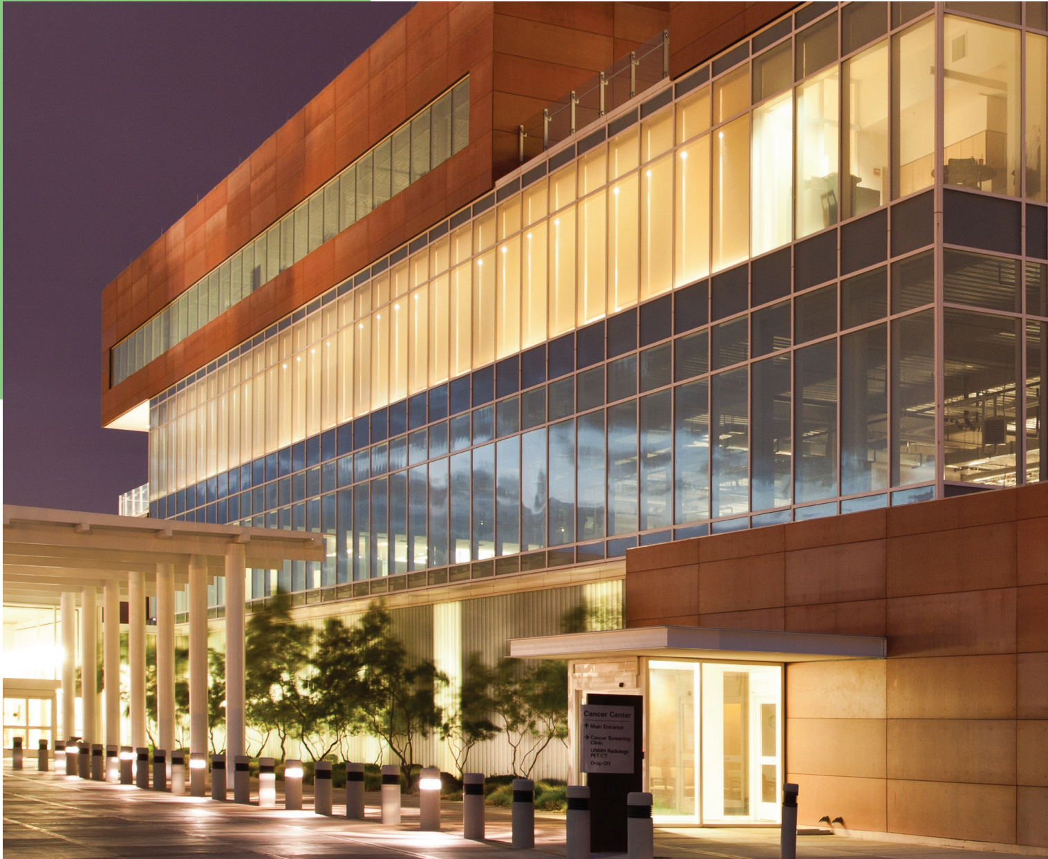
Pictured Above: University of New Mexico Cancer Center, Architect: RMKM Architecture, P.C., Albuquerque, NM Photographer: Matt Oberer, Matt O Photo Albuquerque, NM
